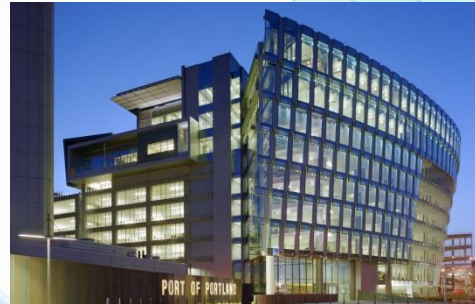
Port of Portland HQ
